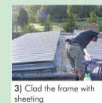
3) Clad the frame with sheeting
