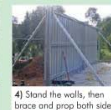
4) Stand the walls, then brace and prop both sides
