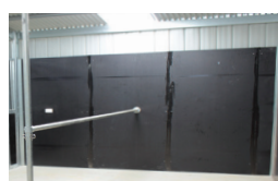
Side Wall with Full Infill in tie up area
